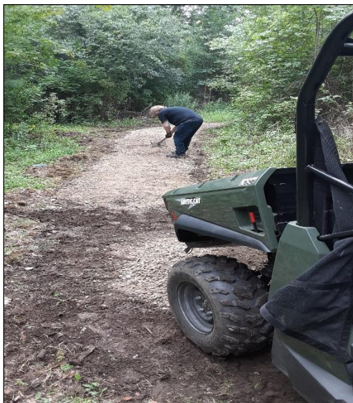
Volunteer helping to build Pond Trail at Raptor Lane
