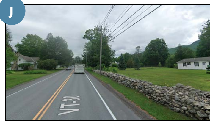
Shift road to avoid ~70 ft of stone wall at 1148 VT 30 (Misai & Misai), currently located within 2 ft of pavement edge.
