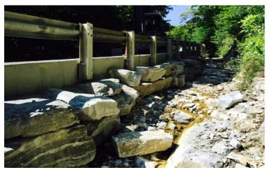
New retaining wall on Lower Squirrel Hollow Road in East Dorset Village. The wall and rocks below are both pinned to bedrock for stability.
