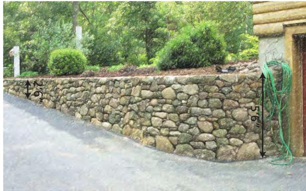
Height measured at point where distance from top of the wall to the ground below is greatest. (ex. wall height = 5'6")
